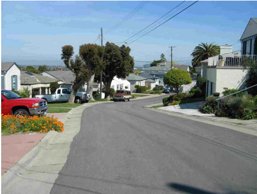
Typical California urban stormwater conveyance system – Street gutter Water & pollutants efficiently moved to creeks
