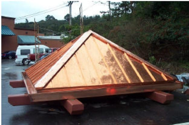
Copper roof section, prior to installation
